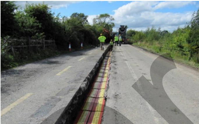
Figure 3.5: Typical HVDC Cable Trench in Road
