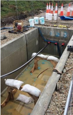
Figure 3.2: HVAC joint bay with one cable pulled
